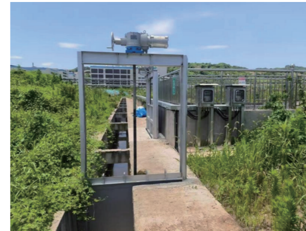
Installation of Online Wastewater Monitoring
