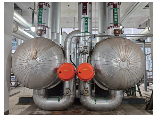
Automation Energy-Saving Retrofit Project for the Ethylene Glycol Loop in the THF Recovery System
