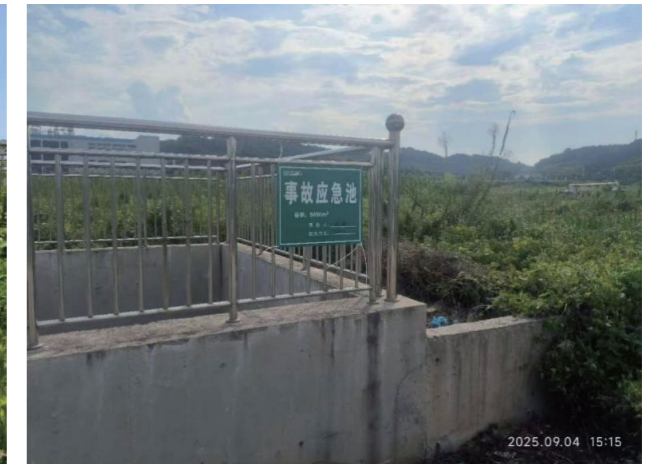
Emergency Basin for Wastewater Discharge Incidents
